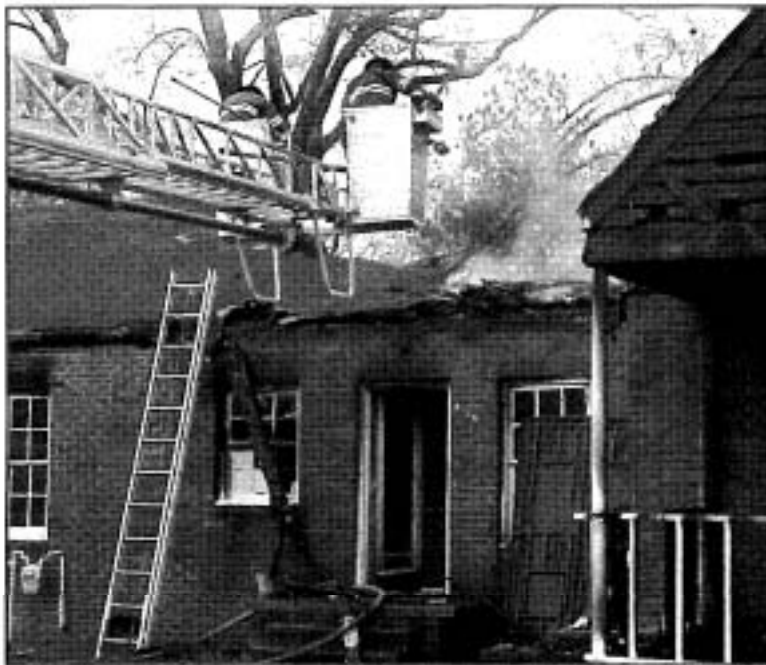
The Chanticleer/Danni Lusk Jacksonville firefighters battle the last remnants of the fire which gutted the Sigma Nu house last month. No one was injured in the blaze, but fraternity members say the house is a total loss.
