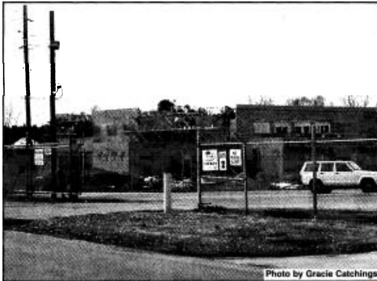
The new Jacksonville community center, as it is shown under construction at Union Yarn Park
