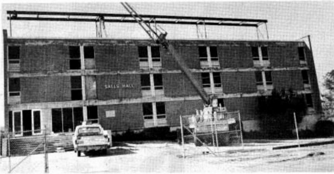
Salls Hall in the early stages of renovation
