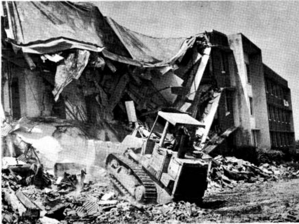
Patterson Hall is demolished
