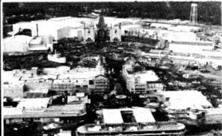
COMING ATTRACTION -- Construction continues on the movie park portion of The Disney-MGM Studios. Buildings along Hollywood Boulevard take shape in the foreground. The theme park's thoroughfare leads to the familiar Chinese Theater landmark and The Great Movie Ride. The Studios, third major gated attraction at Walt Disney World, will open in May 1989. (Copyright 1988 THE WALT DISNEY COMPANY)
