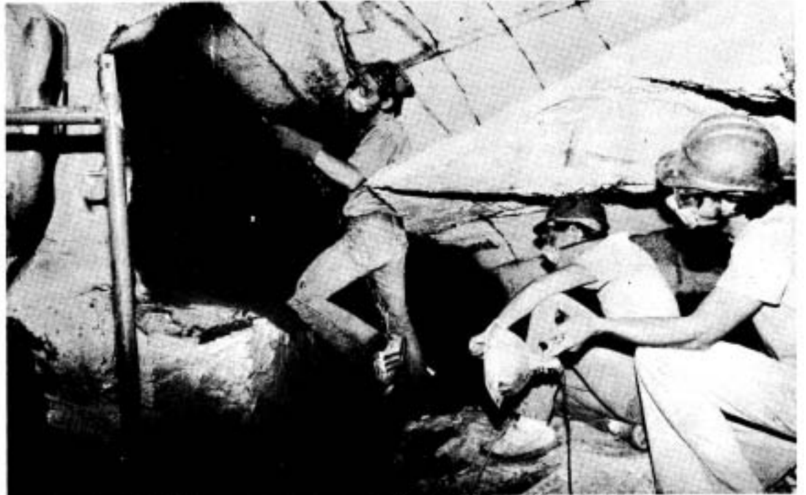
Workers prepare the artificial cave
