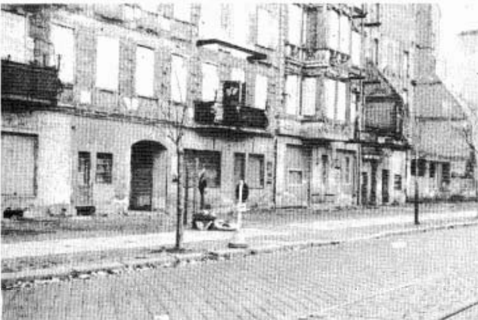
BRICKED UP BUILDING —This building connects two parts of the Berlin Wall. The windows and doors were bricked up to prevent escapes.
