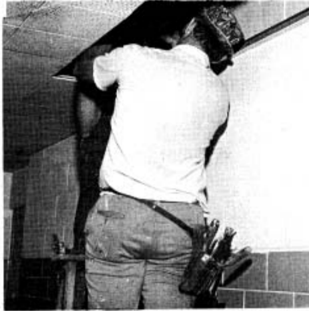
Workman installs air conditioning.
