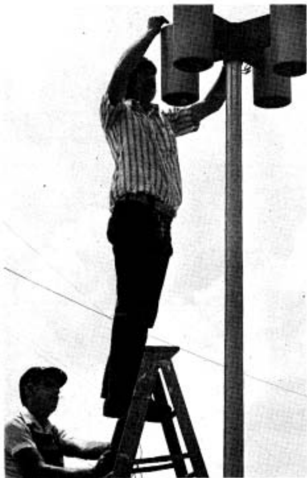
Workmen prepare lighting at Salls Hall for fall semester.
