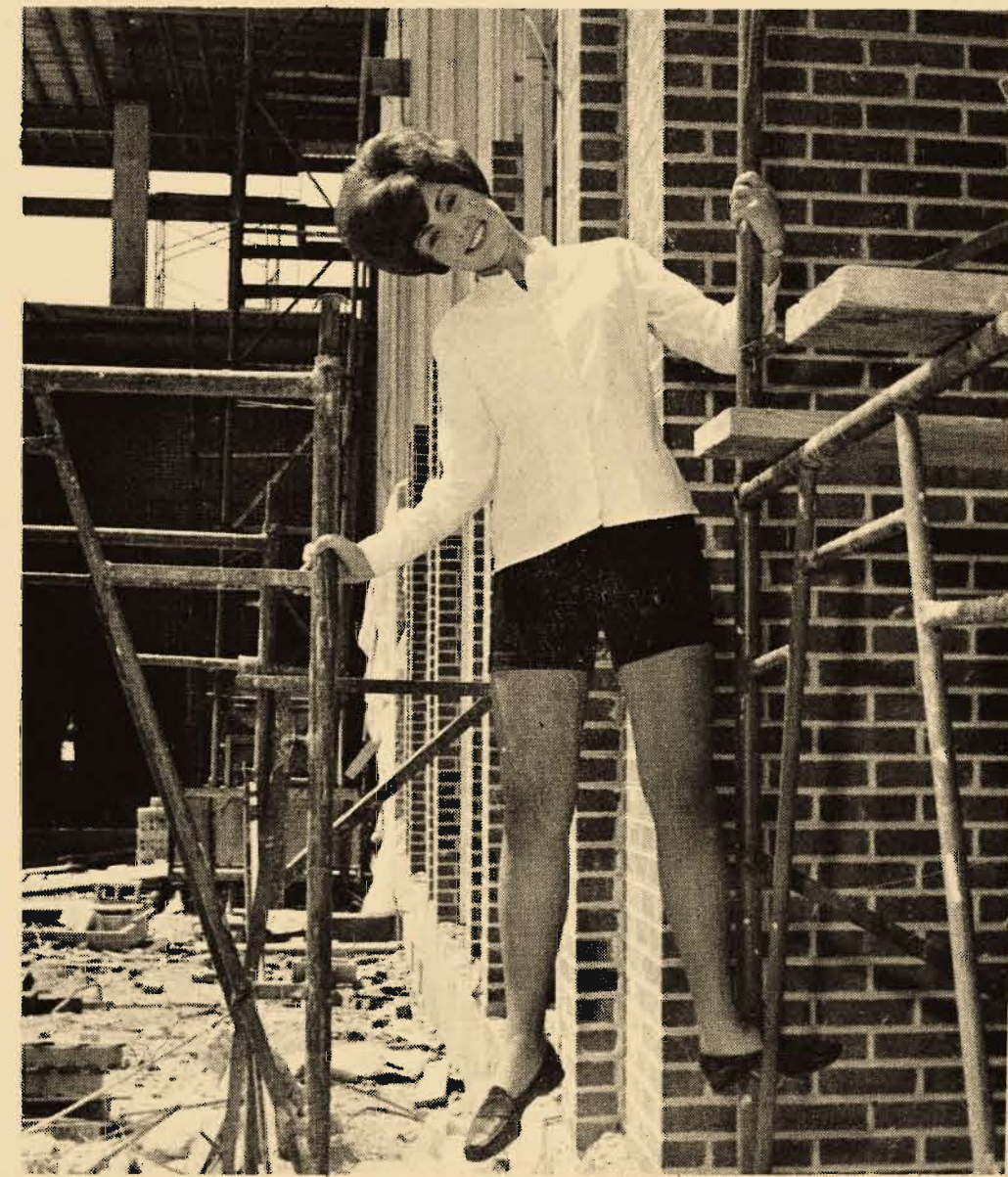
Lovely Sharon Kramer of Gadsden monkeys around the construction site of JSU's newest classroom building. If she stays around there very long, you can bet your life that the workers will never finish the building.
