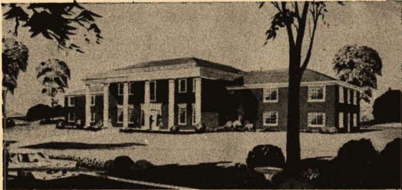
INTERNATIONAL HOUSE--Now under construction.... The new International House will be ready for occupancy this fall.
