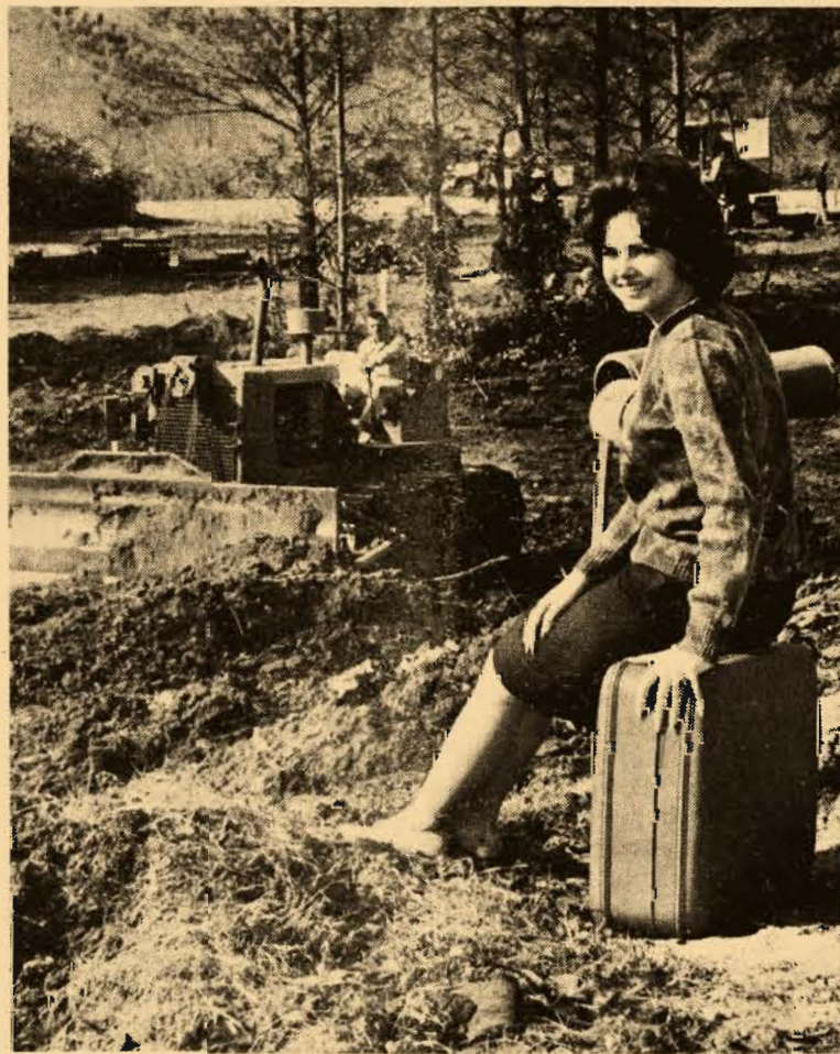
GEM OF THE HILLS—First on the waiting list for a room in the new girls' dormitory is pert and pretty Jo Ann Thrasher, who patiently watches excavation of the construction site. Our eager beaver is a freshman from Gadsden.
