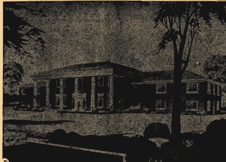
BREAK GROUND — Pictured at right are officials of the International House Foundation who recently broke ground for the new International House. They are, from left, Col. C. W. Daugeette Jr., Mrs. A. C. Michaels, Mrs. Edwin D. King, and Col. H. M. Ayers. Pictured above is the architect's design of the proposed building.
