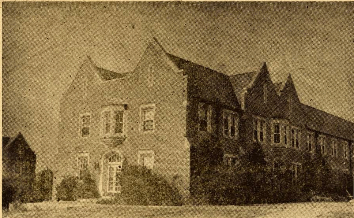
ABERCROMBIE HALL —The first dormitory for boys on the new campus was erected in 1939 when Dr. C. W. Daugette served as college president. It was named for the late Dr. John Abercrombie, one of Alabama's most renowned educators, and was originally an apartment dormitory. It is now directed by Miss Lucille Branscomb.
