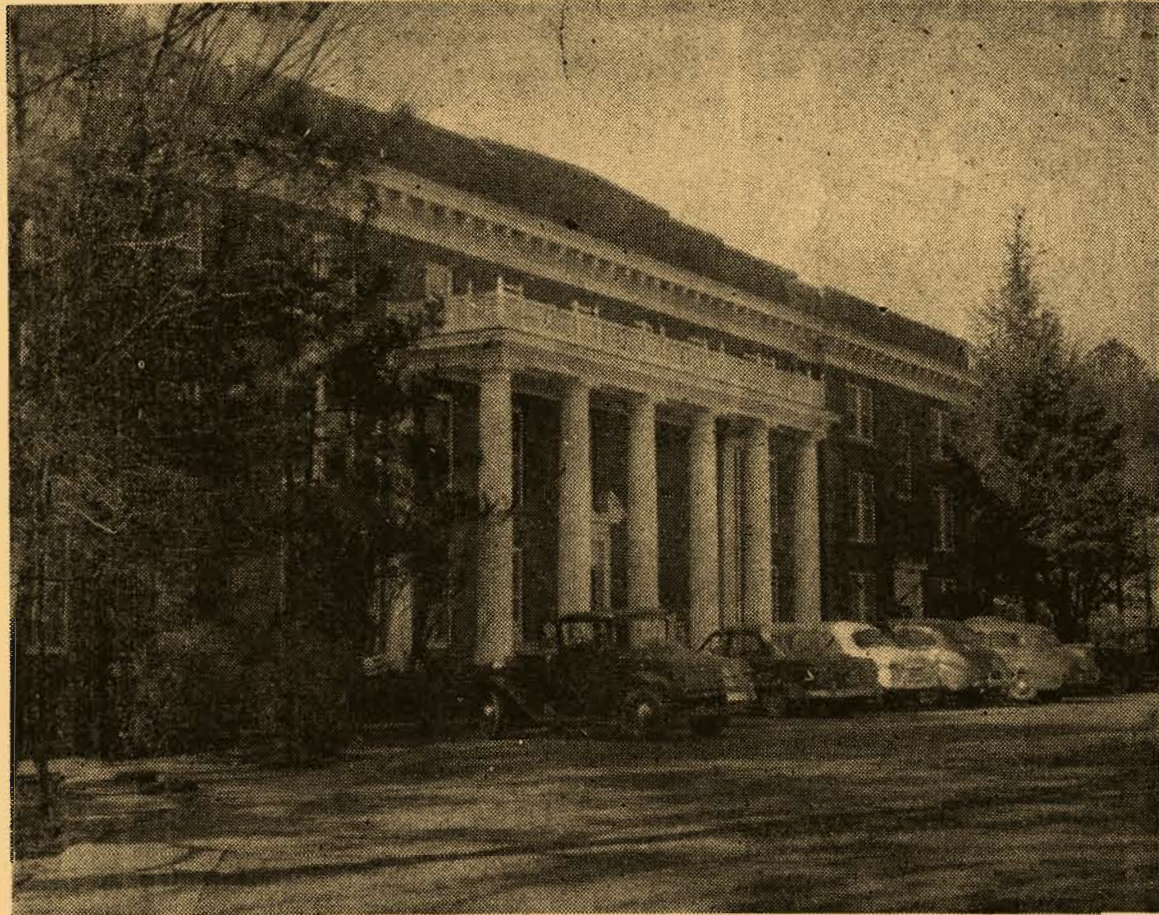
JACKSONVILLE LANDMARK —Forney Hall, erected in 1927, stands as a monument to the old State Normal School here. The building, named for Gen. John H. Forney, is used as a boys' dormitory.
