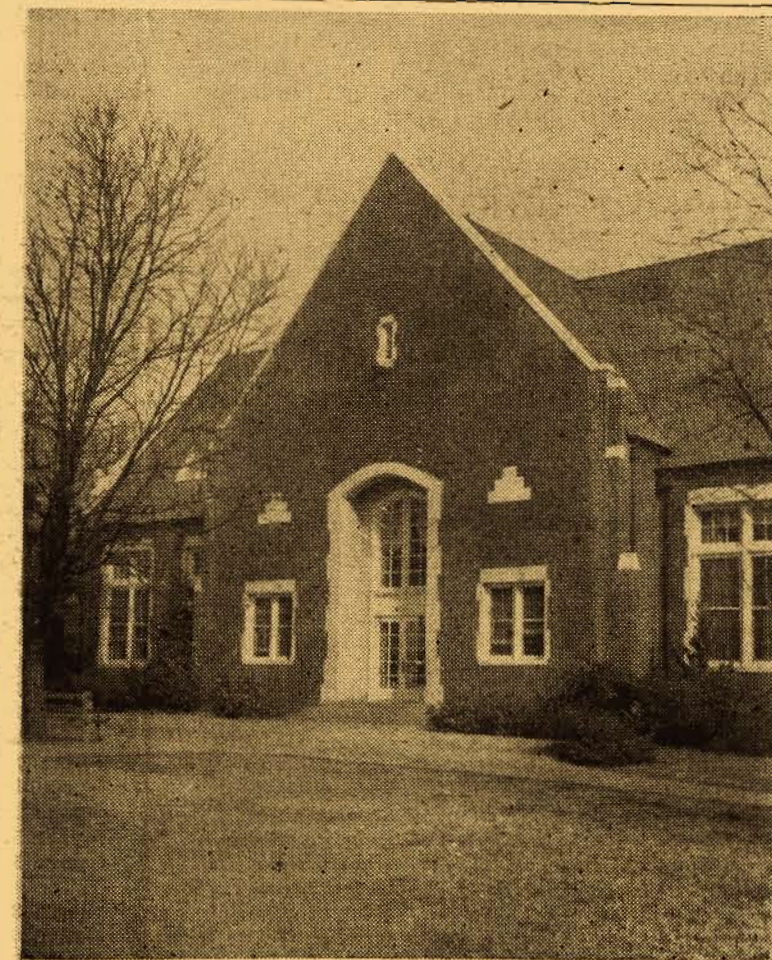
DINING HALL—dormitory hall, located next to the Administration building, is the student cafeteria.
