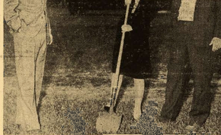
Pictured above is Miss Carolyn Triplett, a popular co-ed, who is breaking the sod to launch a building expansion program at J. S. T. C. The photo was made on the site of the wing to be added to the north-west corner of Daugette Hall at an estimated cost of $200,000. The contract was awarded to Jones and Hardy Construction Company of Montevallo, Alabama. Lumber, steel and other building materials have appeared on the scene, and the excavation has already begun.
