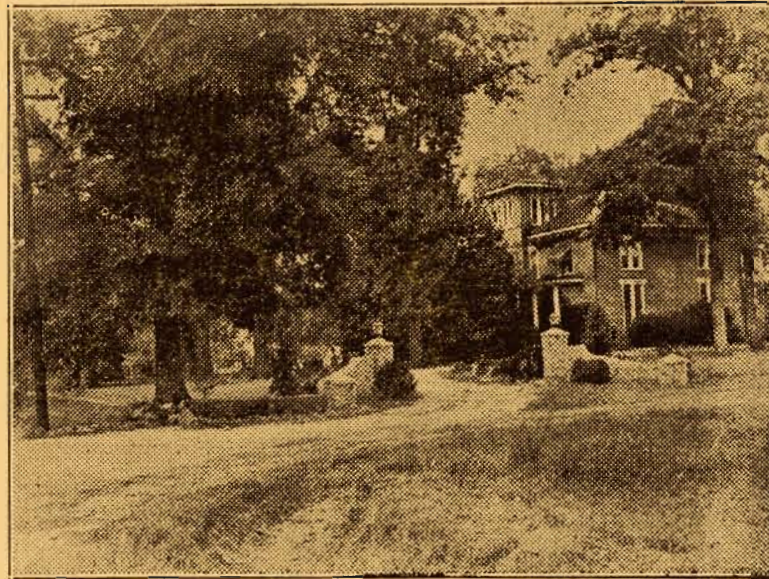
"The Magnolias", home of Dr. and Mrs. C. W. Daugette, on North Pelham Road. The home was built by Judge T. A. Walker sometime before the War Between the States. It is of brick construction, with high ceilings and spacious rooms. The bricks were hand pressed and sun dried and made with slave labor on the spot where the college tennis courts are now located.
