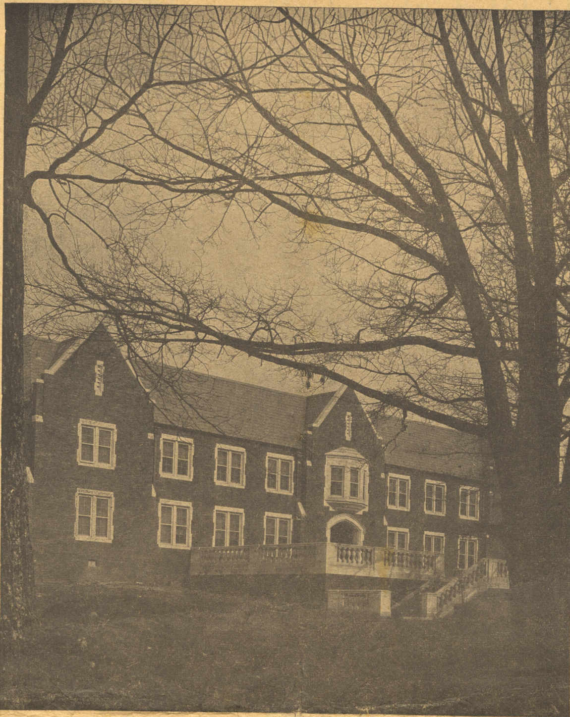
DAUGETTE HALL A fire-proof Dormitory for Women
