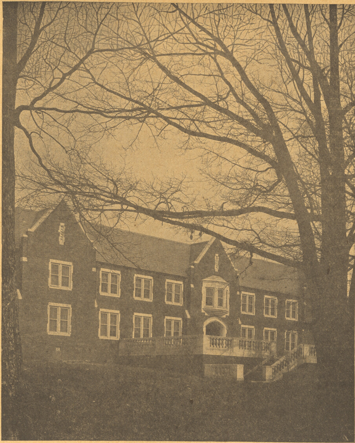
DAUGETTE HALL A fire-proof Dormitory for Women
